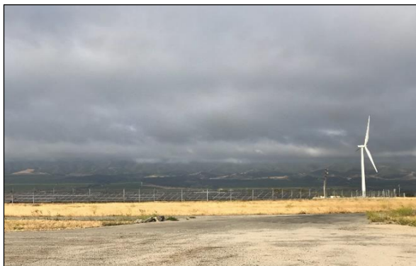
Figure 16- Wind Turbine and Solar - CTF
