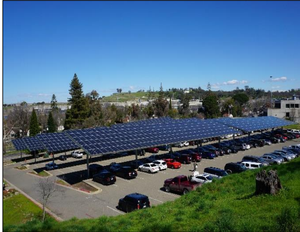
Figure 15- Solar Canopy System – CSP-SAC
