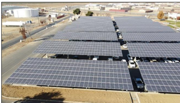
Figure 2- Solar Parking Canopy Installation at VSP
